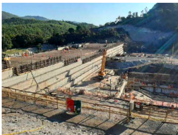
Figure 10. RCC containment dam below Sul Superior.
