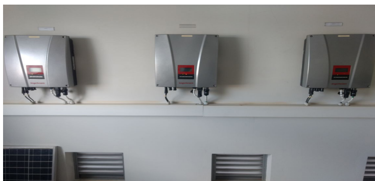
Figura 4 – Inversor INGETEAM modelo Ingecon Sun Lite 3,68TL
