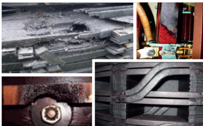
Figure 3: Fault examples (from the left to the bottom: D2,D1, T3 and T1) (CIGRE - JWGD1/A2.47, 2019)
