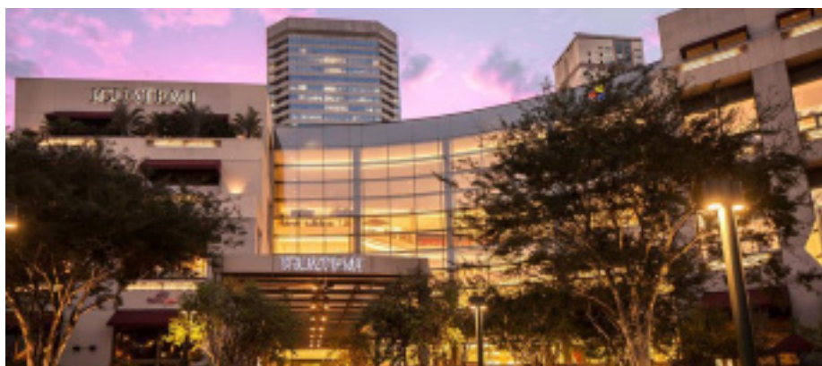
Figura: Fachada do Shopping Iguatemi Alphaville, 2019.
