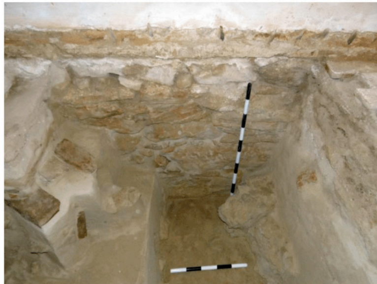
Figure3–Note the foundation with unmortared juxtaposed stones.
