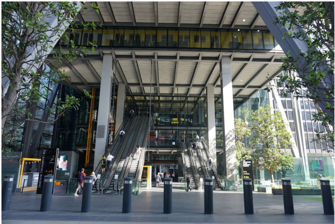
Figura 7: Térreo permeável do Leadenhall Building .
